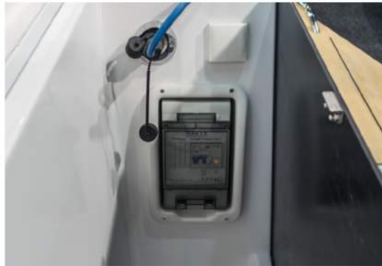
Shore Power 230V with 40Ah charger
