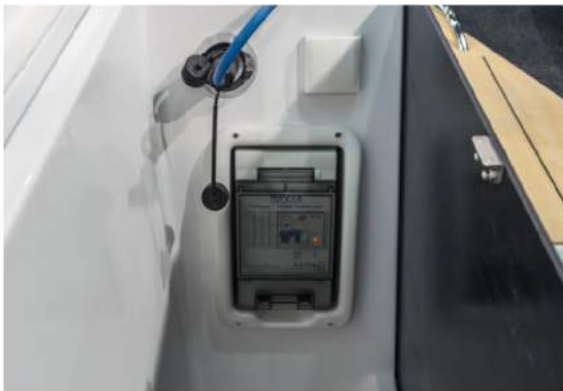
Shore Power 230V with 40Ah charger
